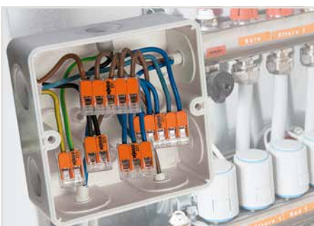
Wiring fine-stranded conductors in a junction box.
