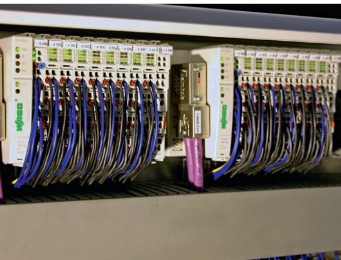
1. Decentral PROFIBUS couplers exchange data between the controller and the sensors and actuators.
